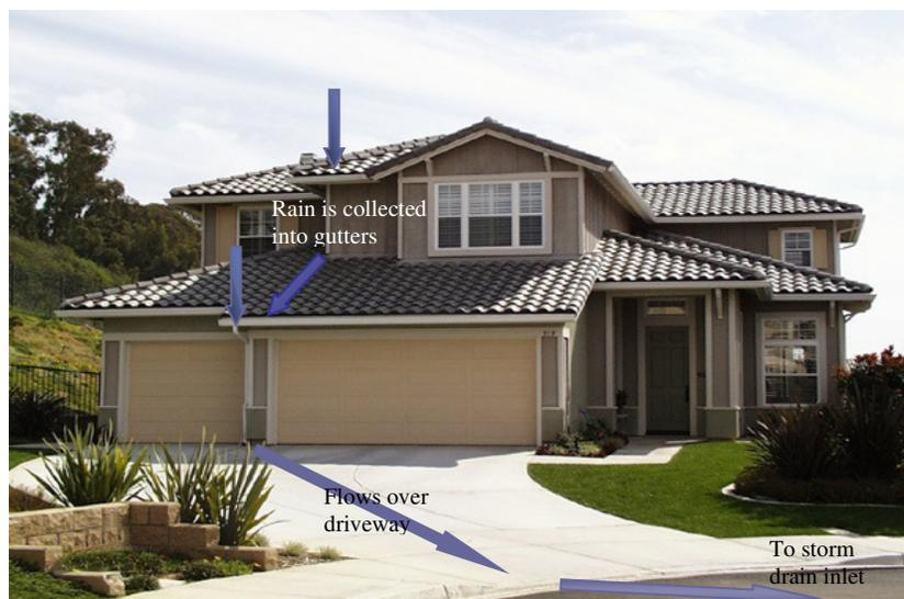
Rainwater is intercepted by roofing and collected into gutters. The water then discharges the downspout onto a paved driveway and flows to the gutter and storm drain inlets. Alternatively, the collected water is piped underground directly to the storm sewer.
